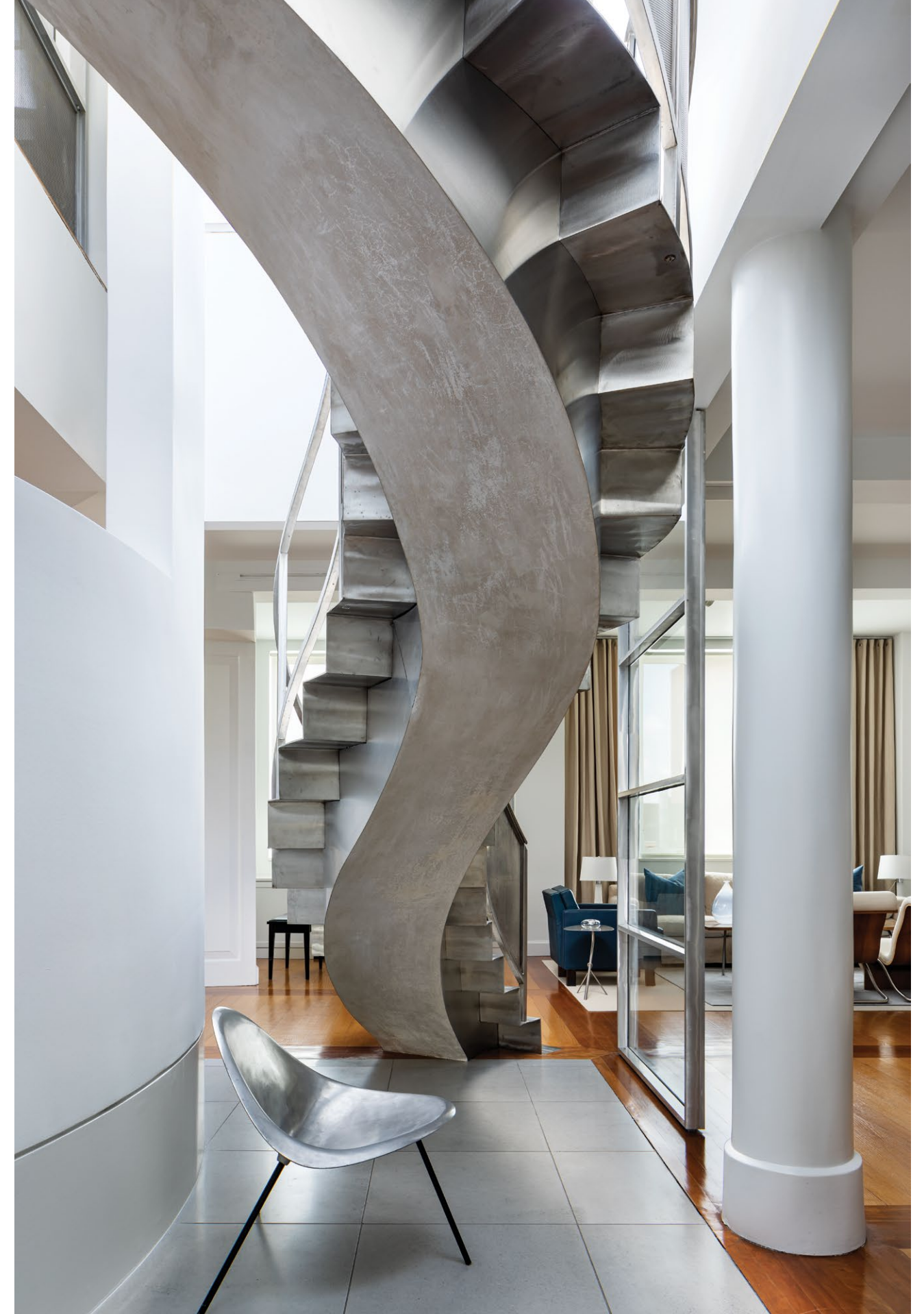
Stainless steel and concrete double helix staircase / Stainless steel chair: Poul Kjærholm prototype, DMK. (Opposite page) Meeting space: ceramics by Amsterdam artist Wouter Dam, Galerie VIVID / prototype table by Tom Dixon. Photos: Michael Moran/OTTO
